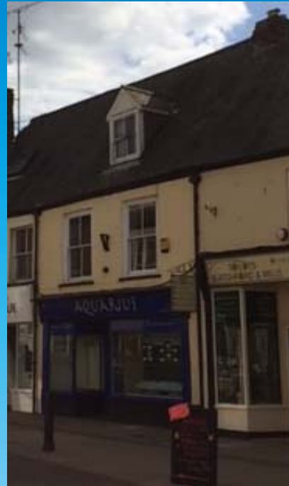
8 Tower Street Before
